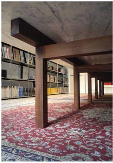
Constructed of timber posts and beams and fitted with thick slabs of marble, the table is built as one would erect a temple. Basic teakwood frames are joined with spanning members using simple pegs at the top of each column. The heavy stone is then aligned to rest securely above, completing the primitive structure.
